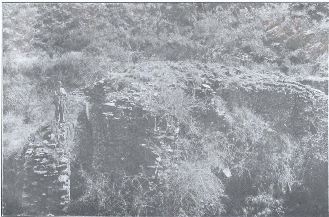
FIG. 11. BROKEN WALLS IN CENTRE OF BARRAGE, TŌKAR-DARA.
